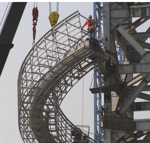
Steel being erected for the theater tower.
